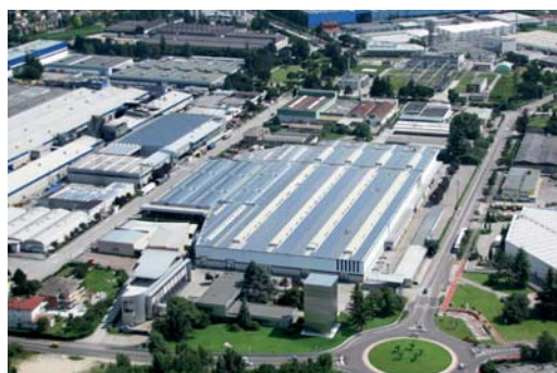
ROVERETO - TN - PREMISES AERIAL VIEW
